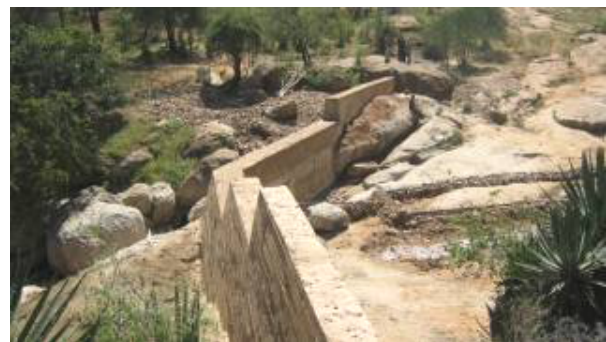
Dam angled to follow the bedrock and bring the flow back to the centre of the river
