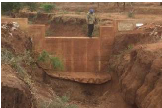
Examples of poorly constructed dam aprons
