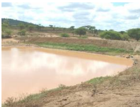
Earth Dam, Kenya. Credit: UDO / EDK
