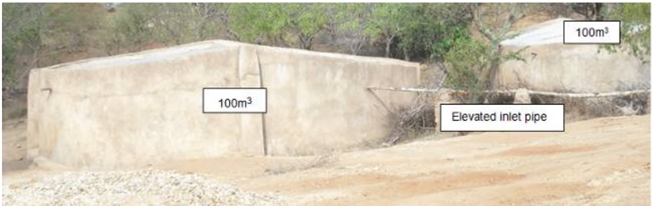
Rock catchment and storage tanks
