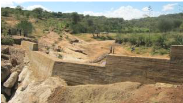
Dam angled to follow the bedrock and bring the flow back to the centre of the river
